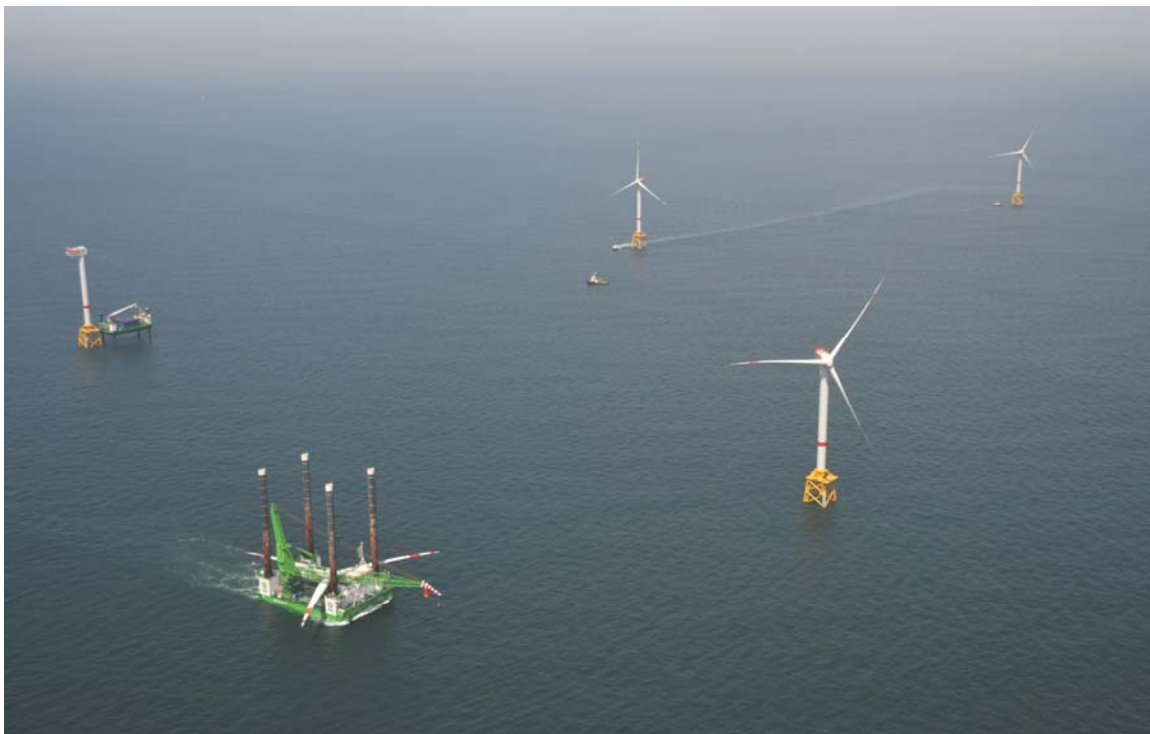
Turbine transport and installation on the Thorntonbank
