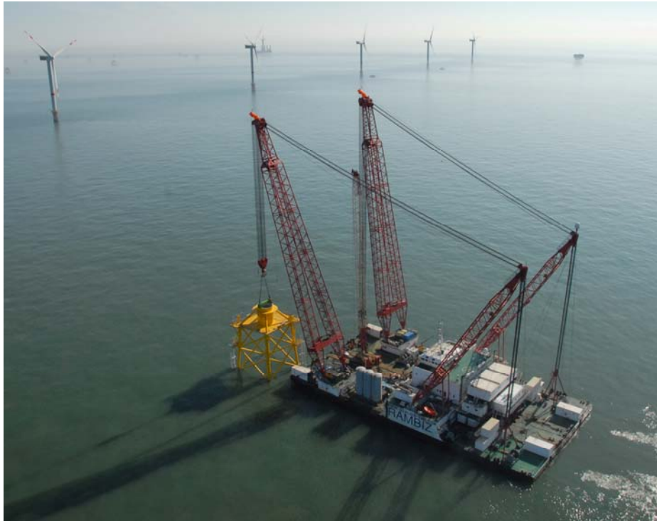
Figure 3. Phase III jacket installation (Photo C-Power).
