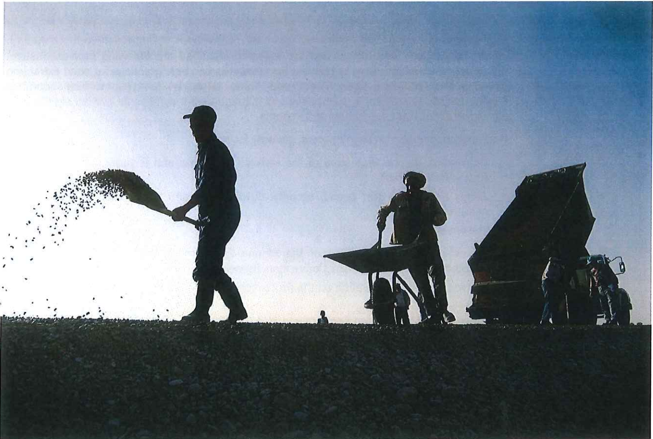
Workers on a road construction site
